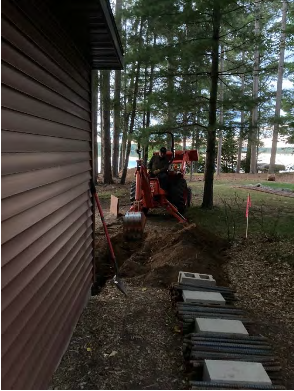
Trenching from pumphouse to lake. Note cut rebar stored near pumphouse.
