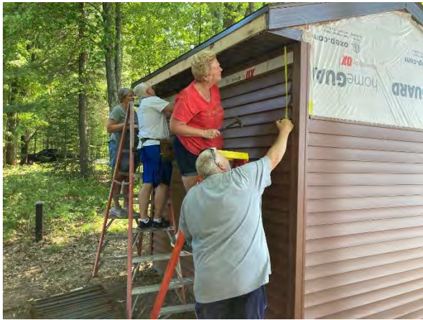
Finishing pumphouse build
