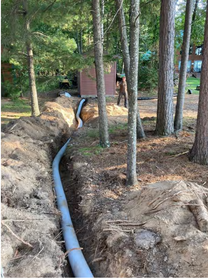
4 pvc airlines encased in 3" pvc from pumphouse to edge of lake
