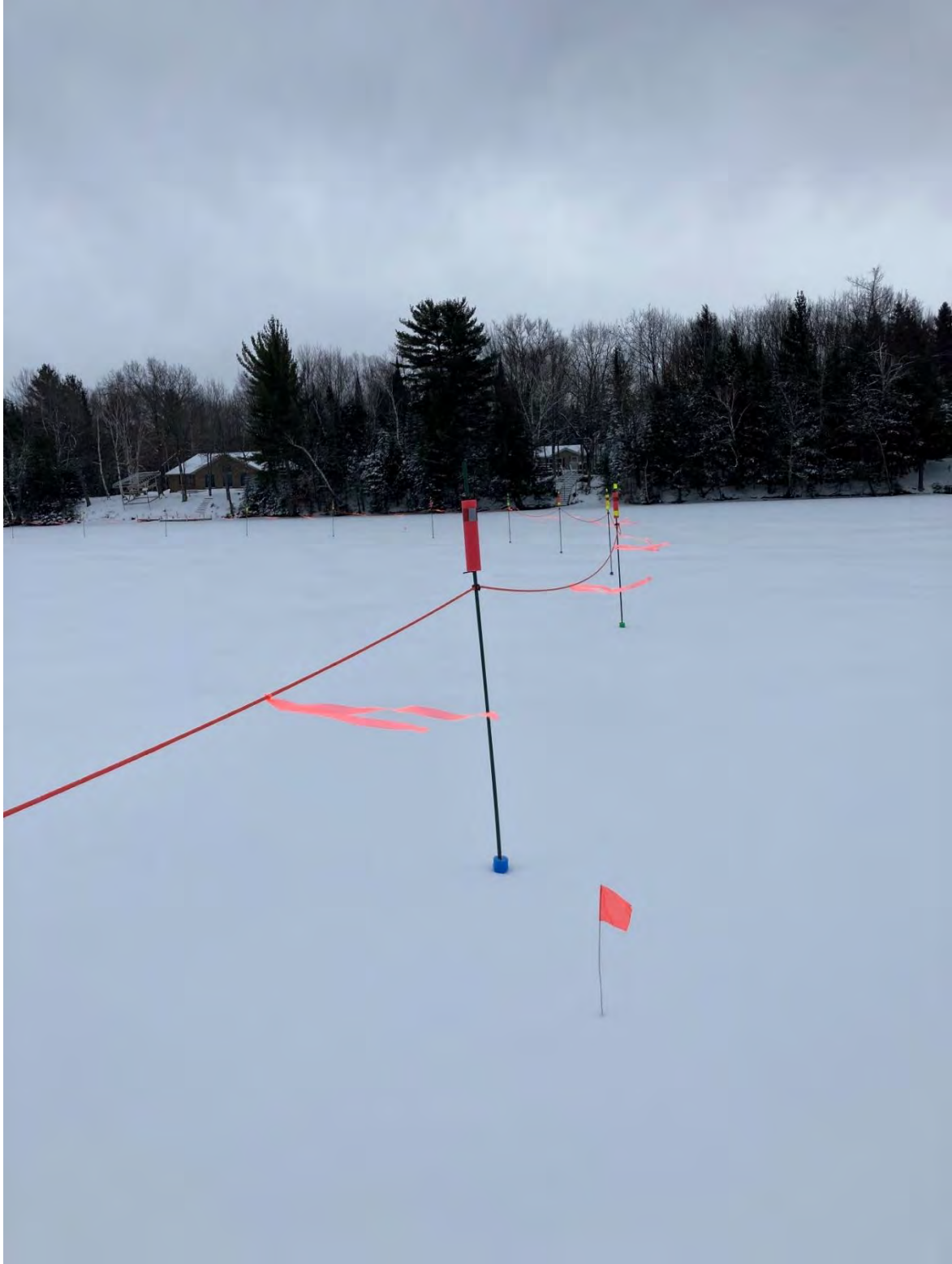
Final barrier install for first season.
