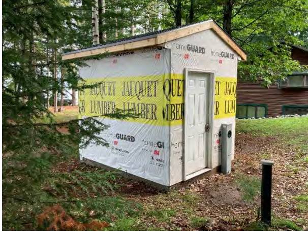
Initial pumphouse build
